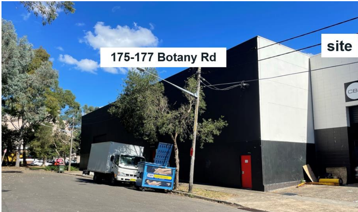
Figure 11: View of site and adjoining commercial development at 175-177 Botany Road fronting Cope Street
