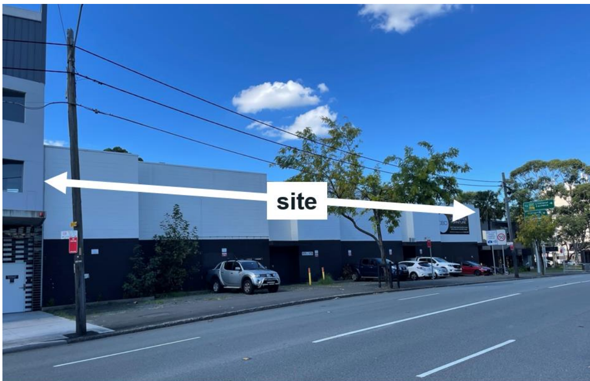
Figure 2: Site viewed from Botany Road
